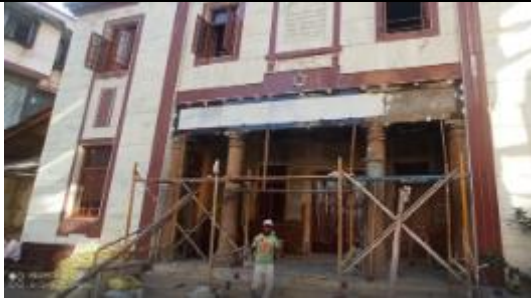
Front beam marble and Granite fixed
