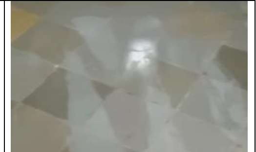
Floor polishing completed
