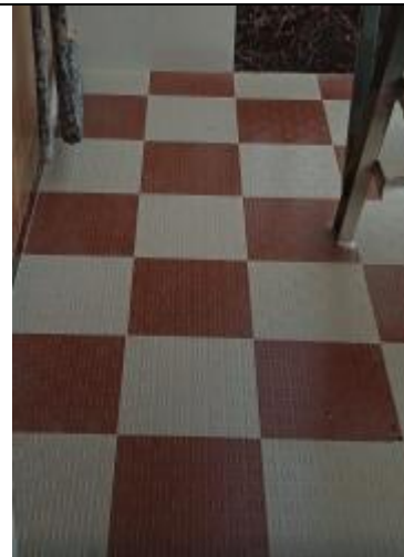
Tiles fixed in staircase gallery
