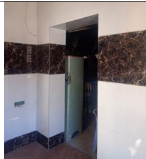
Double vitrified Italian marble pattern tiles fixed in Trustee office
