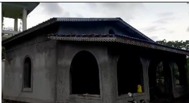
Ambapur Synagogue work in progress
