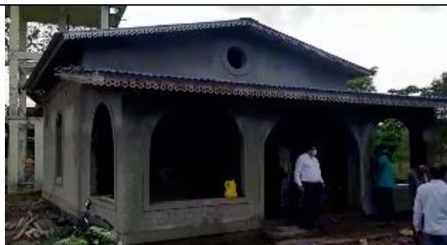
Ambapur Synagogue work in progress
