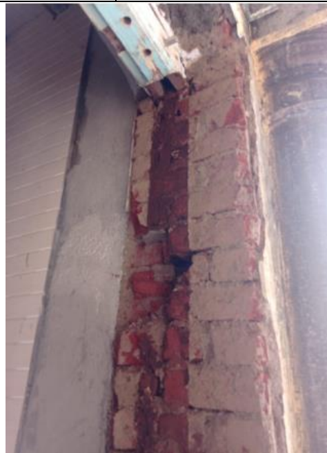
Water seepage on window frames
